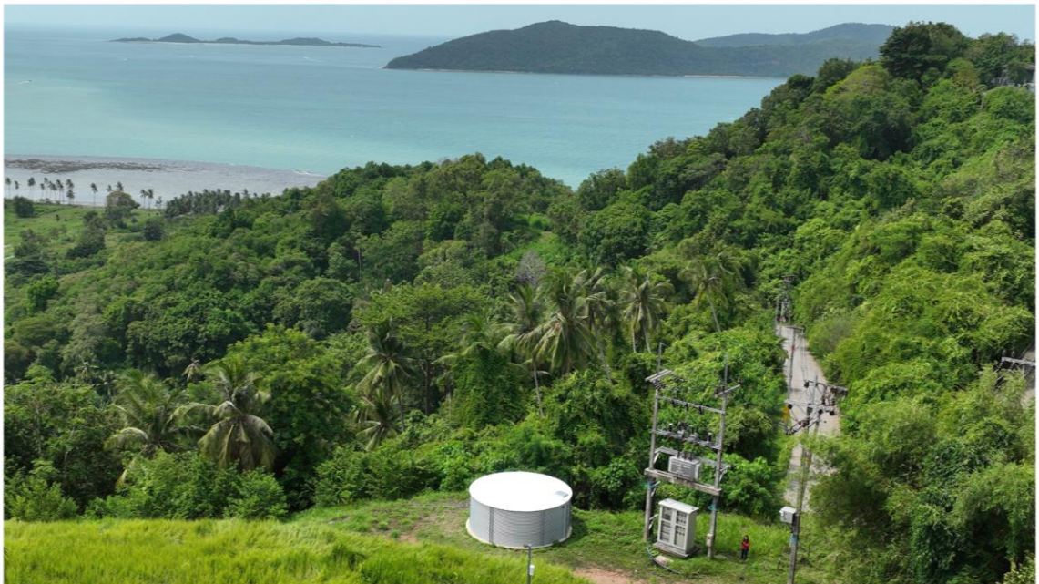
Khun Angkana House RCT60-22 (58,640 liters) Koh Samui Suratthani
