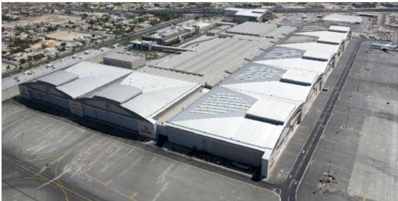
Emirates Engineering Centre, Dubai, UAE. KingZip SF Standing Seam System.
