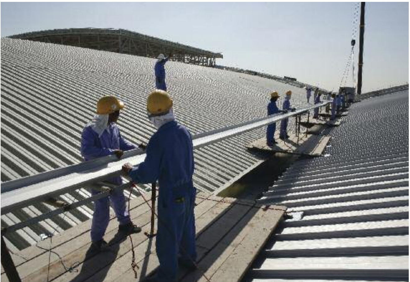
Emirates Engineering Centre, Dubai, UAE. KingZip SF Standing Seam System - on-site roll forming
